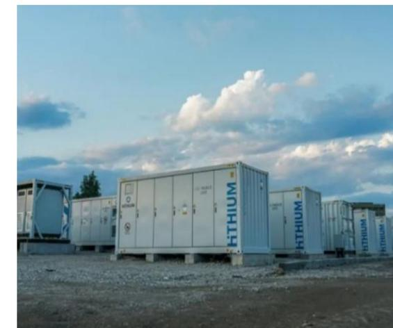
Figure: Hithium ∞ Block Liquid-Cooled Energy Storage System ▶
